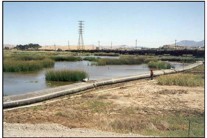
AquaDams® at an oil refinery in Martinez, CA.
