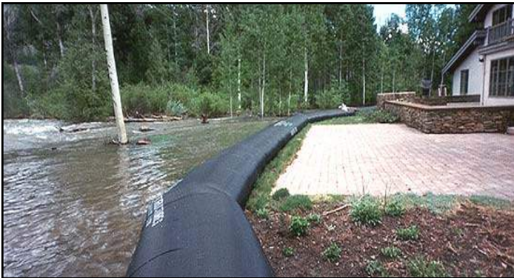
More 3' and 4' high AquaDams® used for flood protection in Sun Valley, ID.
