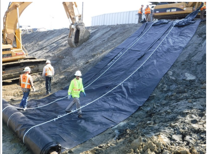
8'x100' long AquaDam has been unrolled down the starting bank.
